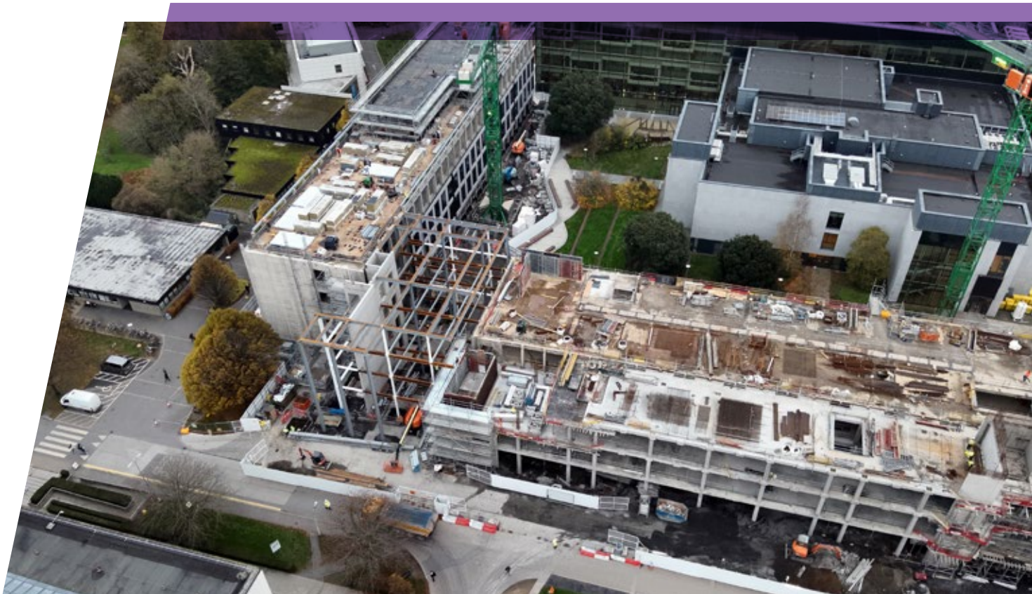
Renovation works continue on Science Phase 3.
